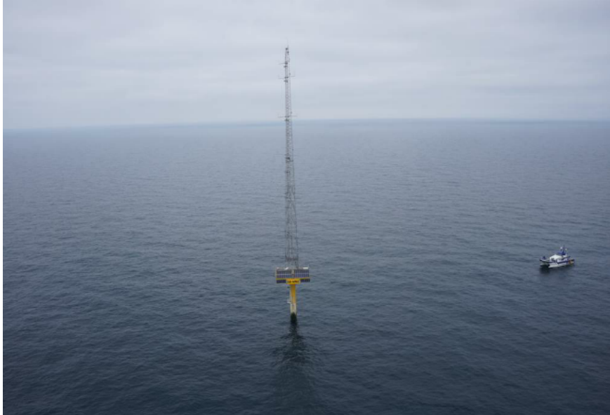
Aerial photo of Dogger Bank Met Mast East and Tidal Transit's Eden Rose taken by Cyberhawk. Source: Forewind
